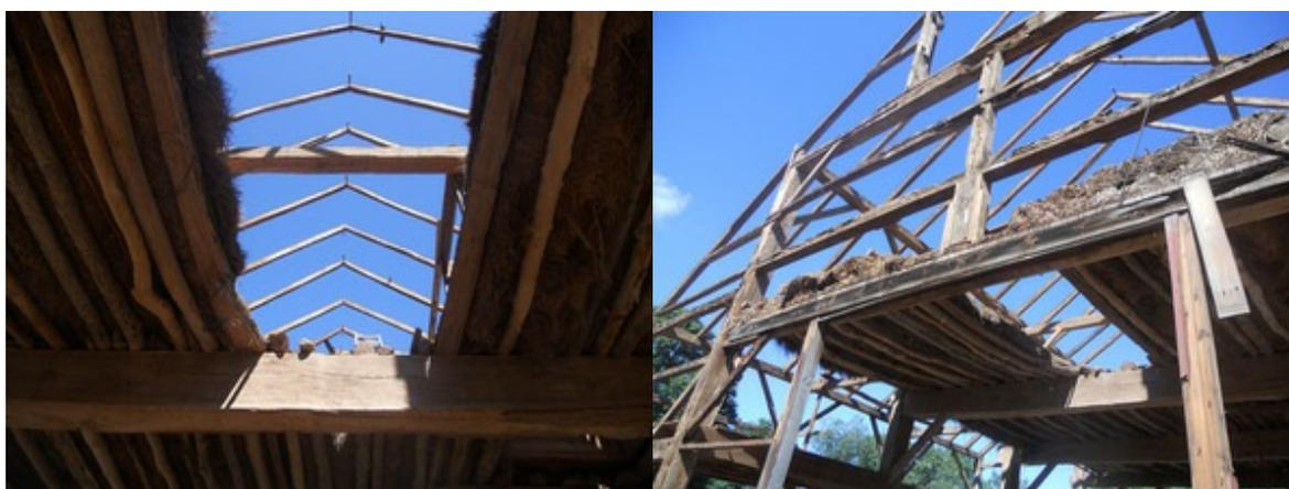
Restoration Technologies then carefully and methodically dismantled the Voorhees Dutch Barn (so-called for a historic owner) in preparation for its repurposed life in Bedminster. The salvaged beams and rafters (primarily composed of oak and poplar), some original hardware, and stone were placed inside a 44-foot trailer and transported to the Vanderveer property where they await reassembly.
